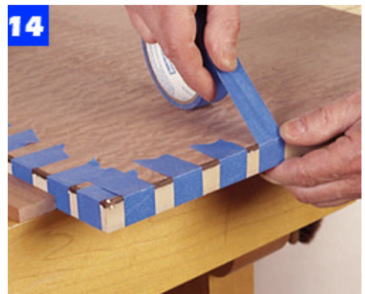
Apply glue to the rabbets and install the inlay. Use tape to clamp the strips in place, and sand or scrape them flush.
